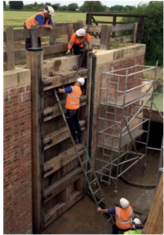
Above: Restoration of Lock 15, Grantham Canal
