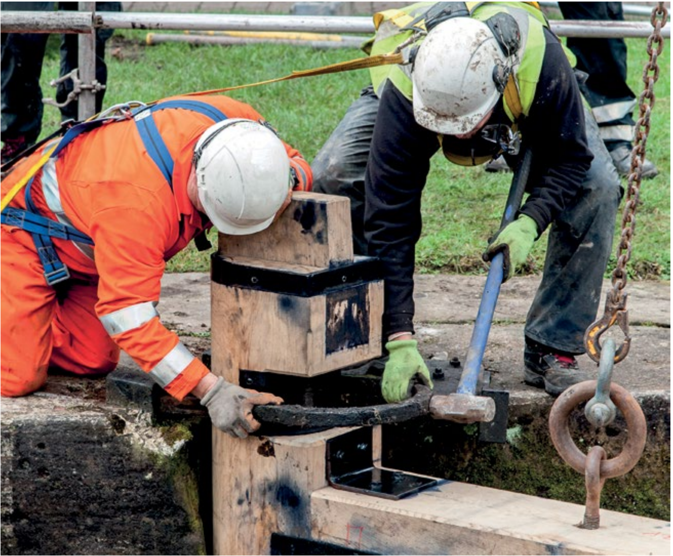
Above: Replacing lock gates
