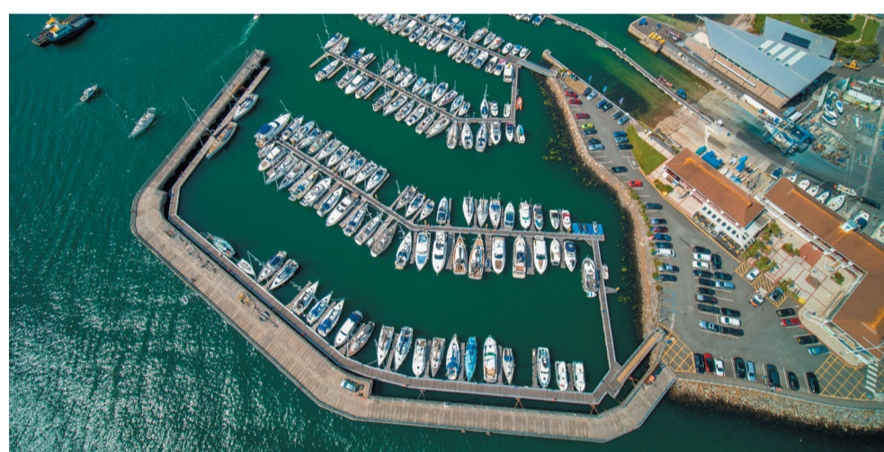
Checking lines, boatfolk Marina, Portland
